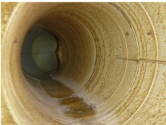
Without ozone cleaning system
