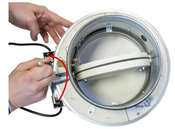
5. Push the fuse back in, keeping the blade in the open position. The shorter tooth of the fuse locks the blade in place.
