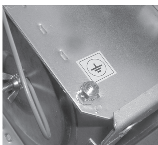
Fig 4. The grounding screw on the fire damper
